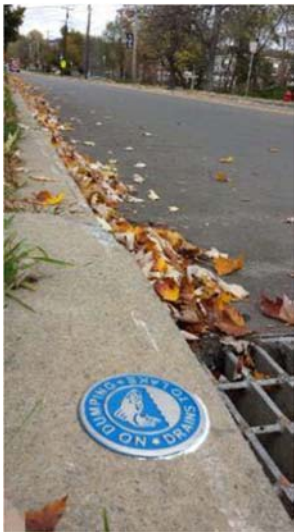
1 Storm drain medallion.
