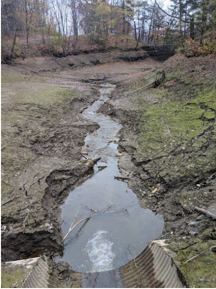
Sediment Retention Basin - Before
