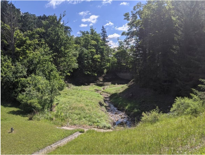
Sediment Retention Basin - After Seeding
