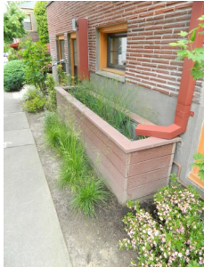
An infiltration planter allows downspout water to slowly permeate into the ground, sidewalk.
