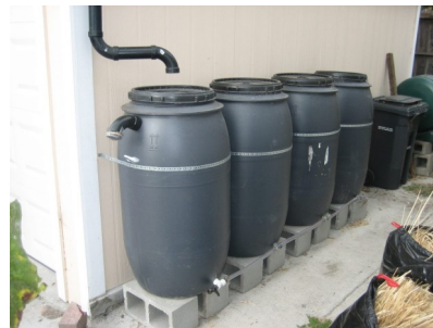
A typical home collection system of daisy-chained barrels, which hold 200 gallons of rainwater.
