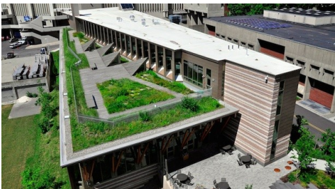
The green roof atop SUNY ESF's Gateway Center. Green roofs also help combat the heat island effect in urban areas and help to insulate the building.
